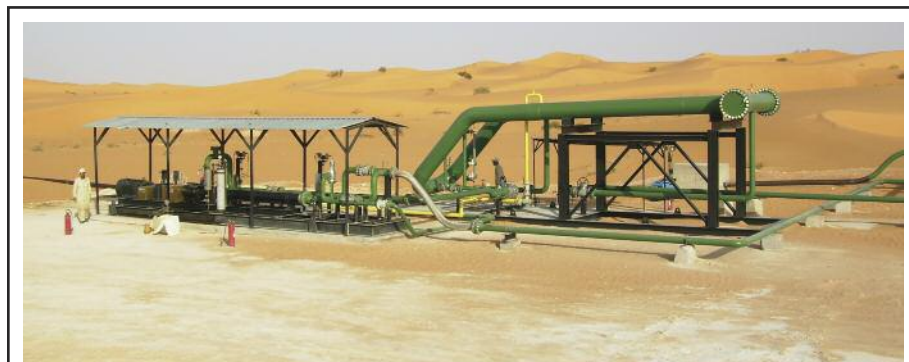
In Algeria, multiphase pumps are being used to produce gas-locked oil wells and optimize flowline pressure to get oil to a central battery, with all pump data monitored from a central control office.
