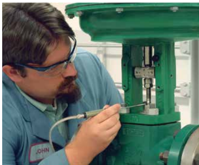
▲ Figure 5. A technician measures the leakage of helium from the packing of a rising-stem valve.
