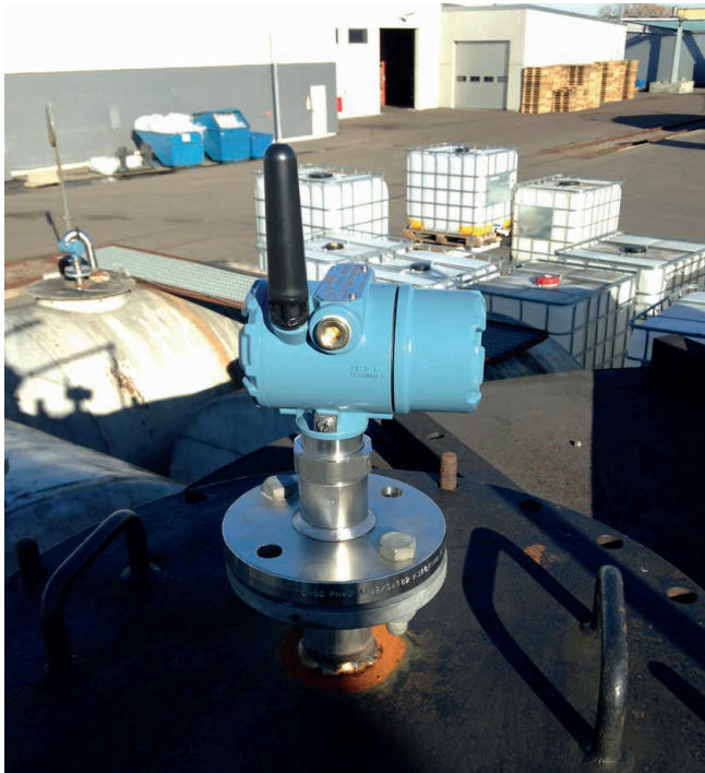
Figure 4. The geographically spread-out arrangement of most tank farms can make adding traditional wired instrumentation prohibitively expensive. Wireless sensors, such as this guided wave radar level device, can use WirelessHART to send information to the automation system.
