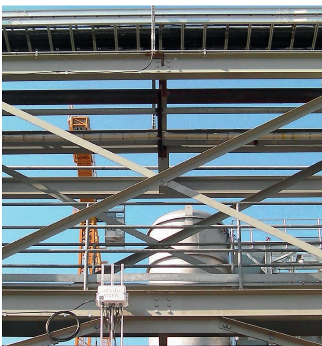
Figure 2. A wireless gateway can serve as backhaul or bridge to other gateways and collect data from many nearby wireless sensors, sending the data to a central computer.
