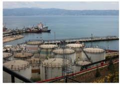
Liquids are landed by tankers at the Altintel jetty, and further pumped into the storage tanks. 50-70 trucks are loaded daily, to provide Altintel's 2200 customers with their product blend.
