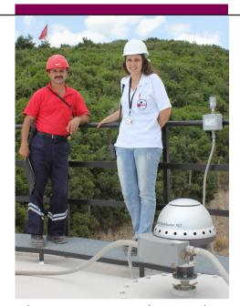
When using automatic tank gauging there is no need for anyone to go on top of the tank. The risk is high, especially during a transfer, when the static electricity in the tank can be as much as 35.000 V. It is a great advantage to watch from a distance.
