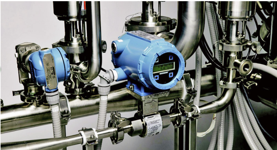
An installed Rosemount 8721 Hygienic Flow Meter
