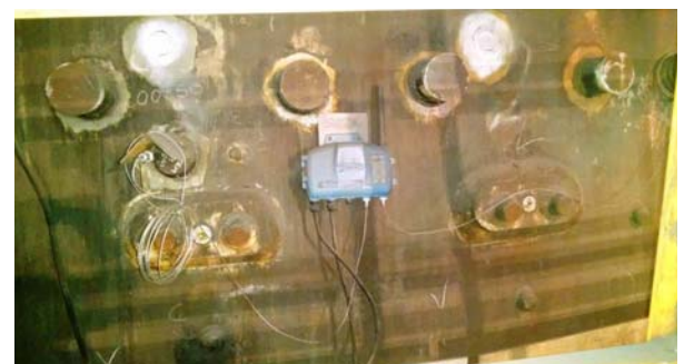
Rosemount 848T Wireless Transmitter installation
