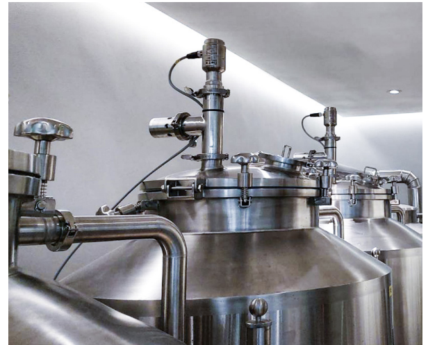
The Rosemount 1408H Level Transmitter was connected to a logic control unit (PLC).
