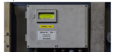
The FLUXUS® G704 CA is used as the measuring transmitter.
