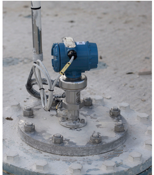
Rosemount 5408 installed in the lime silo.
