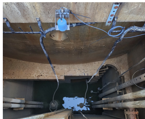
Image #1. The Rosemount™ 1208 Level and Flow Transmitter is installed in a wet well with a mounting bracket.
