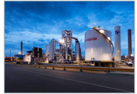
Air Liquide’s air separation plant at Sasol’s Secunda petrochemical complex © Air Liquide
