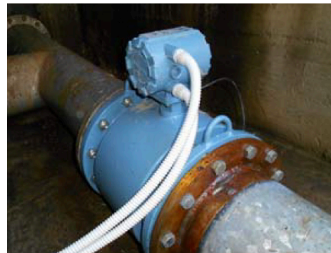
Rosemount Magnetic 10-inch flow meter installed at Mediterranea delle Acque in the filtering area.
