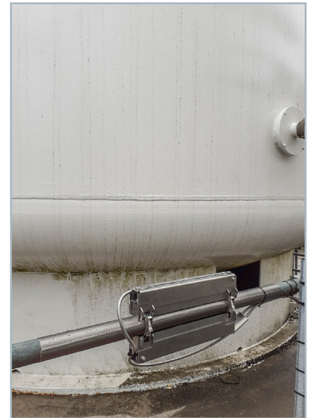
The ideal solution: Continuous oxygen flow measurement from the outside of the pipe.
