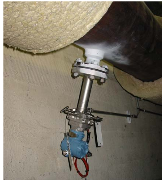
Installation of the Rosemount Annubar Flow Meter
