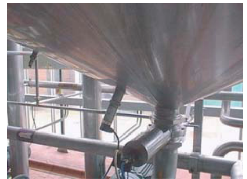
Figure 1. The compact vibrating fork level switch is easily mounted in the bottom of the tank.
