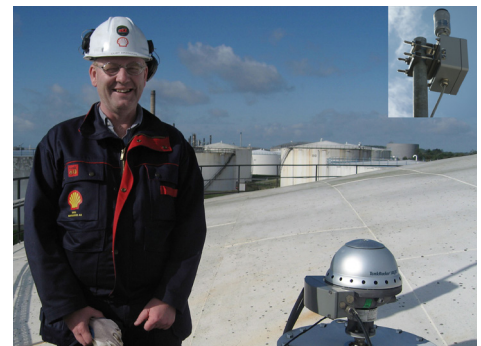
Data from the Rex gauge is sent to the control room via PFN.
