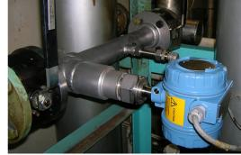
Installation of a Viscomaster meter at the Viscobooster unit (VBU) of the heater control in a ship's engine
