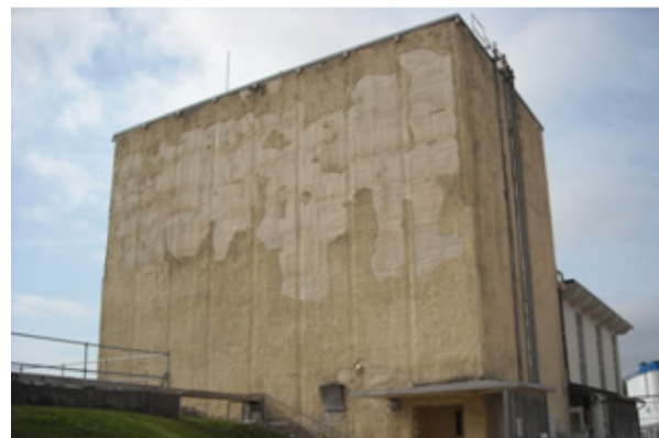
Figure 1. One common building with four quicklime silos.
