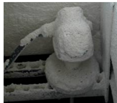
Figure 2. Rosemount 5303 mounted in custom bridge across existing hatch.
