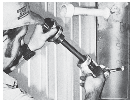
Reseating tool is lowered into valve body after removal of yoke bushing and valve stem.
