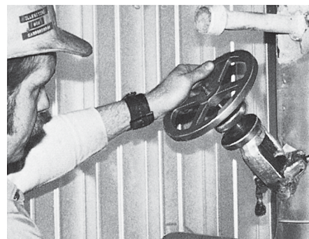
After tool locknut has been tightened against yoke face, to prevent too deep a bite into seat material, seat can be reconditioned by means of a series of five or six slow cuts.
