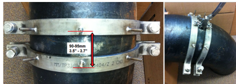
Figure 3-2: Clamp spacing
