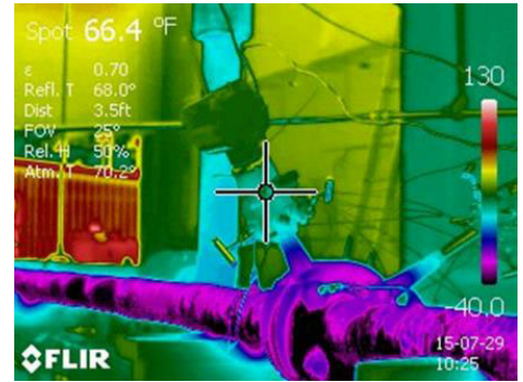
FLIR image of flow meter during cryogenic testing
