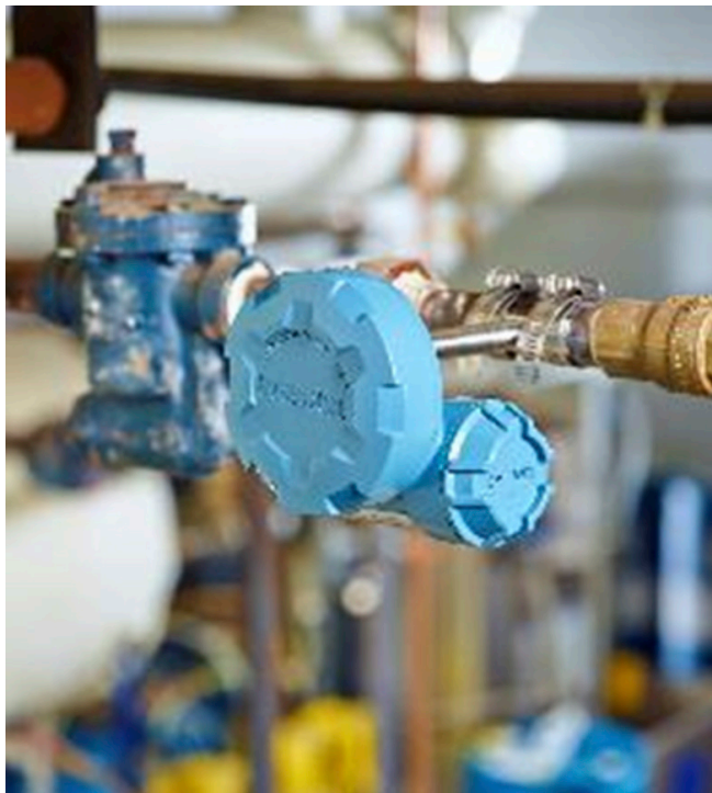
Figure 6. Emerson's Rosemount 708 Wireless Acoustic Transmitter can be mounted adjacent to a steam trap where it listens to its activity and measures temperature. It sends this data to a central collection platform via WirelessHART, so there is no need for wiring.
