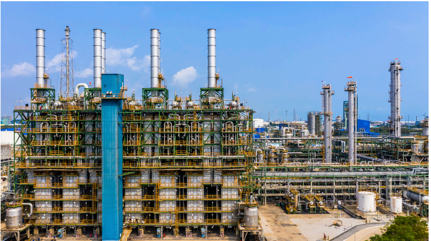
Figure 8. Adding instrumentation to a steam distribution system provides information on consumption patterns to identify steam hogs and other bad actors. Fixing these advances sustainability efforts.
